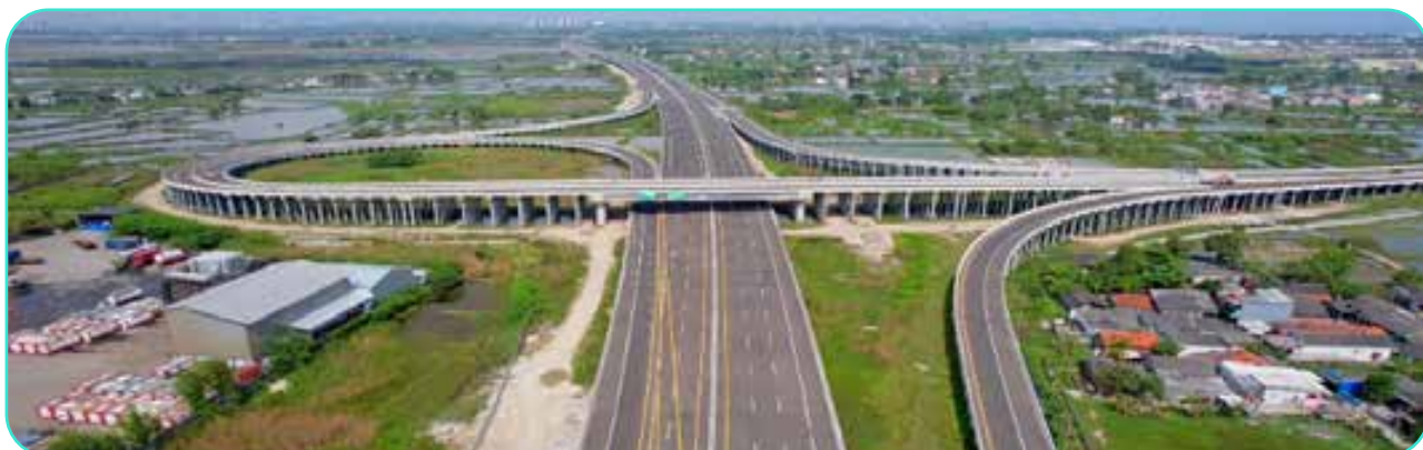
Gambar Dokumentasi Seksi III Jalan Tol Cibitung Cilincing Section III of the Cibitung-Cilincing Toll Road Documentation
