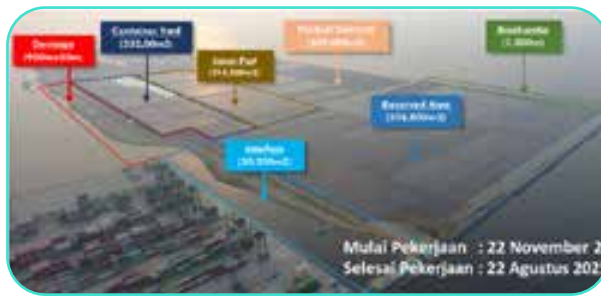
Gambar Progres Pekerjaan Rancang Bangun Terminal Kalibaru Tahap 1B Picture of Kalibaru Terminal Phase 1B Design Work Progress
