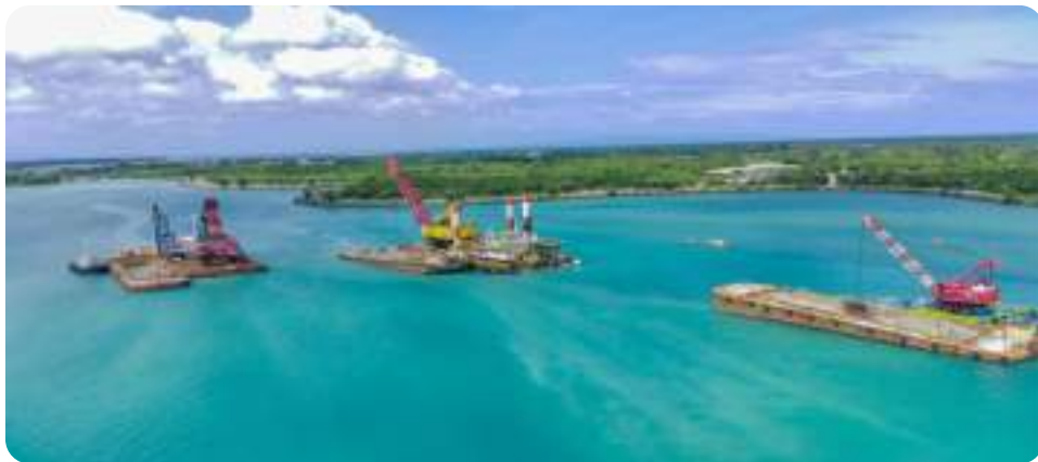
Gambar Pengerukan Alur dan Kolam Paket A Channel and Pond Dredging Package A
