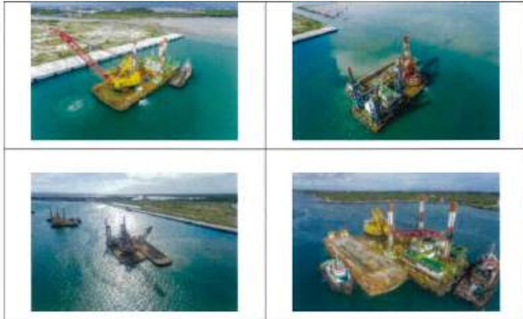
Gambar Pekerjaan Pengerukan di Kolam Dermaga Timur (curah cair, gas, dan petikemas) Photo of Dredging Work at the East Pier Basin (liquid, gas, and container terminals)
