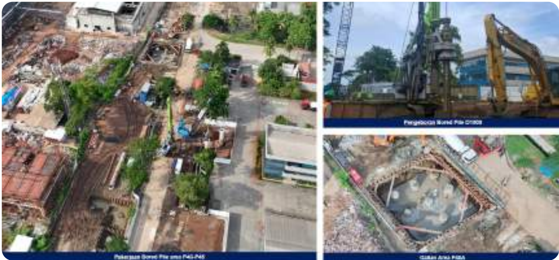
Gambar Pekerjaan Boredpile Area P43-P45 Boredpile Work in Area P43-P45
