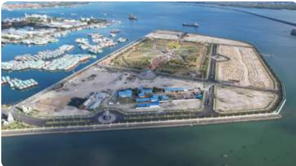
Gambar Pengerukan Alur dan Kolam Paket B Channel and Pond Dredging Package B
