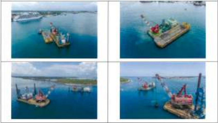
Gambar Pengerjaan Pengerukan Di Kolam Putar Dredging Work in the Turning Basin
