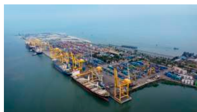
Port of Belawan Capacity: 2 million TEUS
