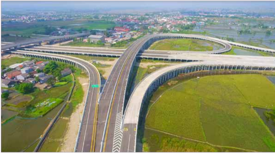
Gambar Progres Seksi III Jalan Tol Cibitung Cilincing Progress of Section III of the Cibitung-Cilincing Toll Road
