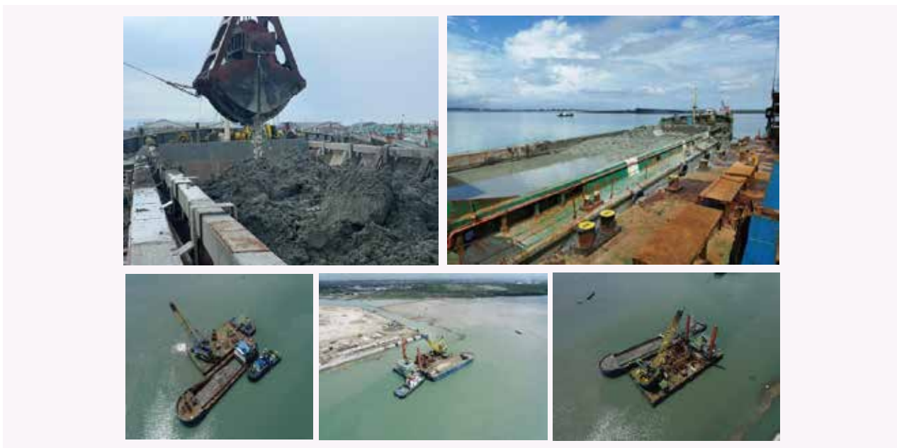
Gambar Pengerukan Area Kolam Curah Cair dan Gas Dredging of Liquid and Gas Bulk Pool Areas
