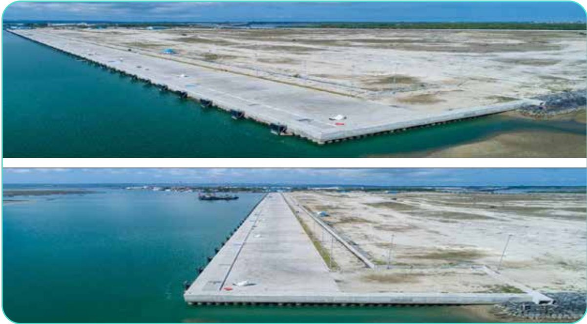
Gambar Dokumentasi Pekerjaan Revetment dan Retaining Wall Dumping 2 dan Dermaga Curah Cair Revetment Work Documentation and Retaining Wall Dumping 2 and Liquid Bulk Jetty
