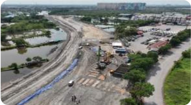
Gambar Pekerjaan Persiapan berupa Timbunan Platform dan Lapisan Geotex Preparatory Work in the Form of Platform Embankments and Geotextile Layers
