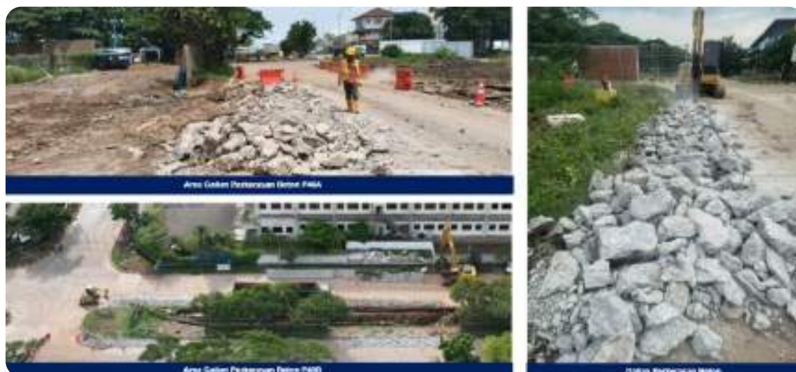
Gambar Pekerjaan Galian Area P43-P46 Excavation Work in Areas P43-P46
