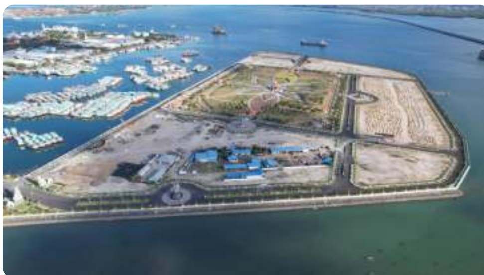
Gambar Pengerukan Alur dan Kolam Paket B Channel and Pond Dredging Package B
